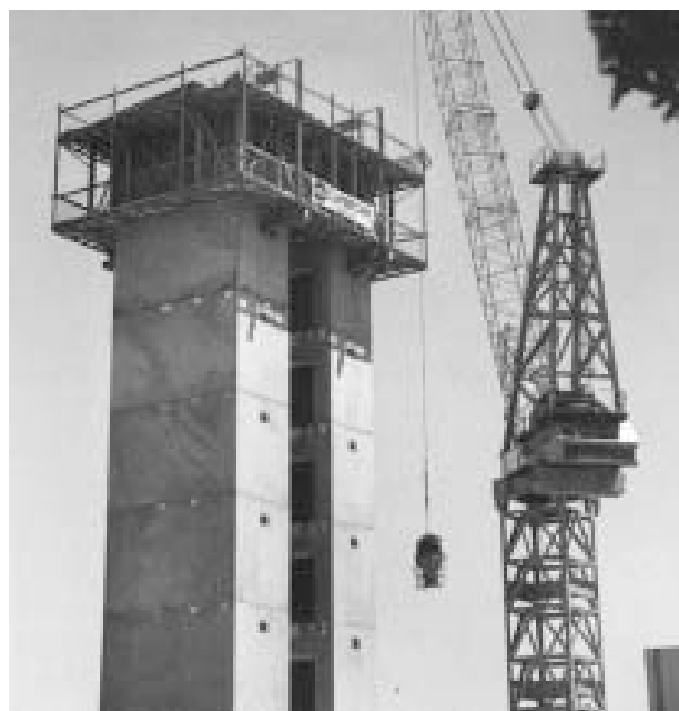
Figure 15.7 Typical self-climbing formwork system
