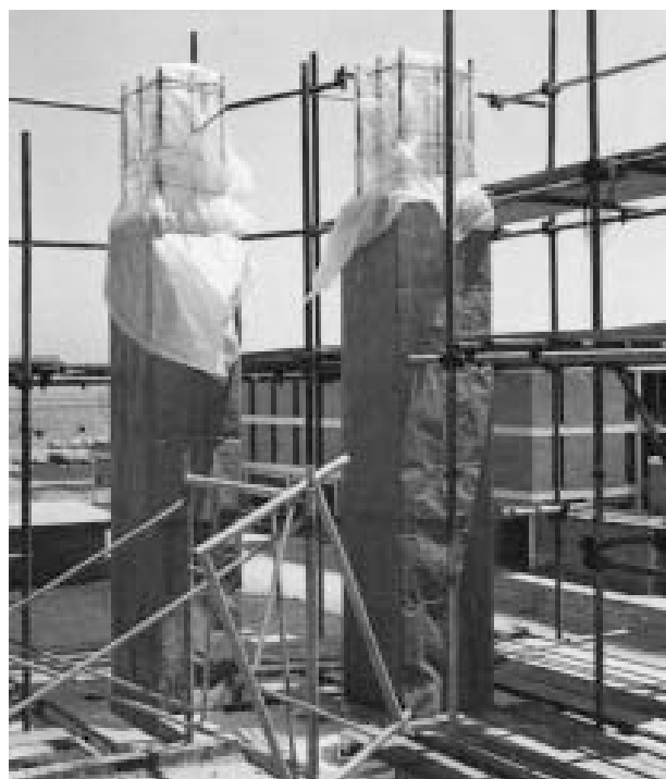
Figure 13.6 Completed work and projecting reinforcement protected by wrapping in building paper and plastic sheeting respectively
