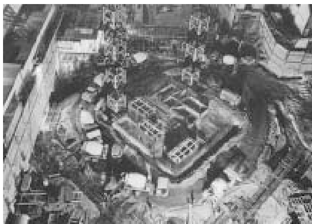
Figure 8.2 Access to the site (and particularly the ease with which delivery vehicles can move on and off it) has a significant influence on the overall concrete supply rate
