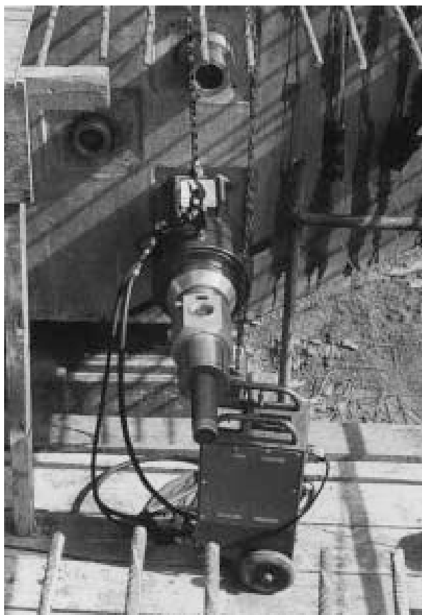
Figure 17.9 Typical hydraulic jack (with hydraulic hoses from compressor unit in foreground)
