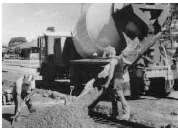
Figure 8.3 Delivery from a transit-mixer chute is the quickest, most convenient and economical method of distribution
