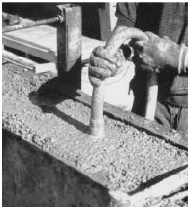
Figure 9.3 Use of an immersion vibrator
