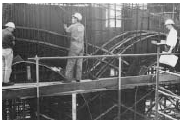
Figure 17.8 Positioning the ducts in the formwork
