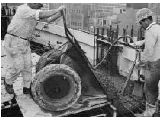
Figure 8.6 Small handcarts (of about 100-litre capacity) have been largely superseded by more efficient methods
