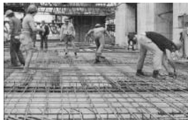
Figure 16.3 Reinforcement being tied in position
