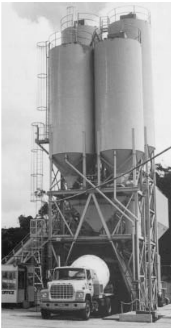
Figure 6.1 Typical medium-sized concrete batching plant
