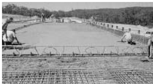
Figure 10.1 Typical trussed vibrating-beam screed
