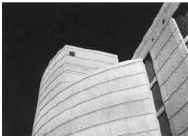
Figure 13.5 Example of bold treatment of tie-bolt holes (and the use of a ribbed finish which disguises minor defects)
