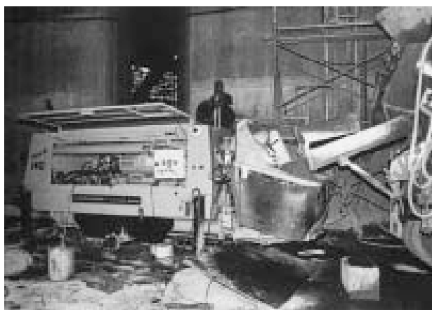
Figure 8.10 Fixed pumps generally have the highest pumping capacity and are the usual choice for major projects
