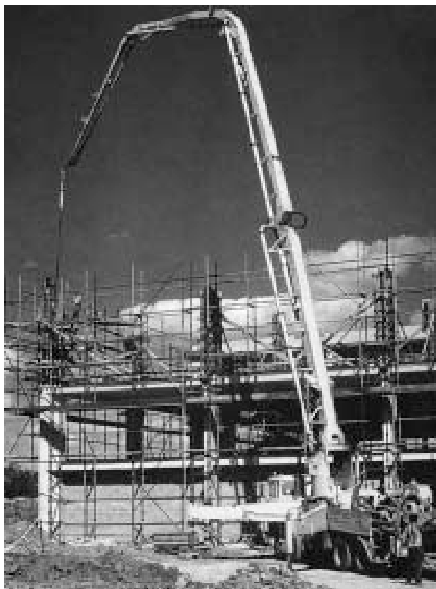
Figure 8.11 Mobile concrete pumps are quick to set up and versatile in their range of applications
