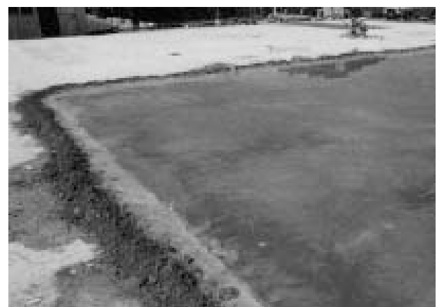
Figure 11.9 Ponding method of water curing
