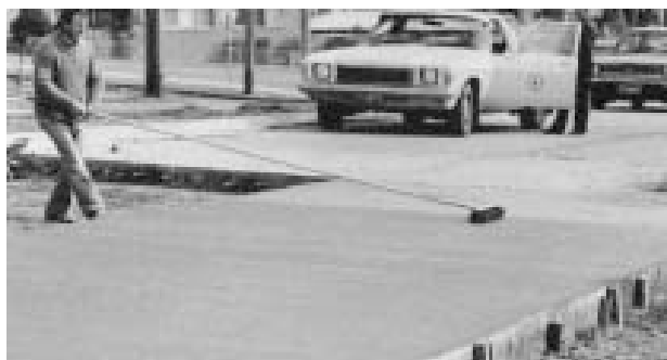
Figure 10.7 Broom finishing to provide skid resistance
