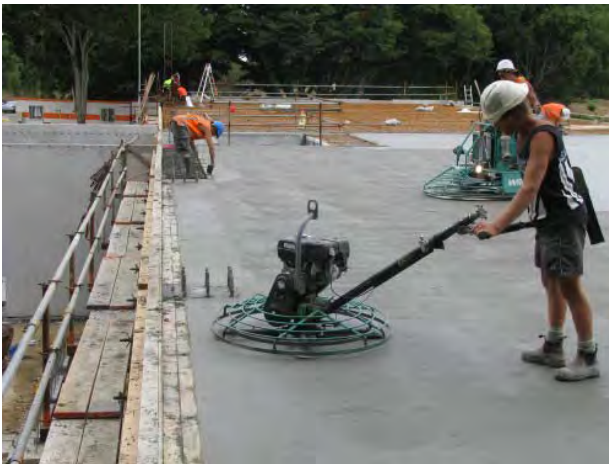
Figure 10.5 Power floating in a regular pattern
