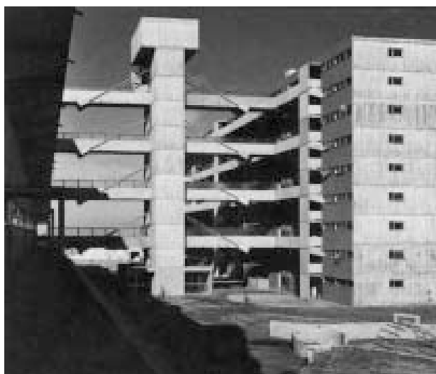
Figure 13.1 Hydration staining resulting from variable absorbency of formwork
