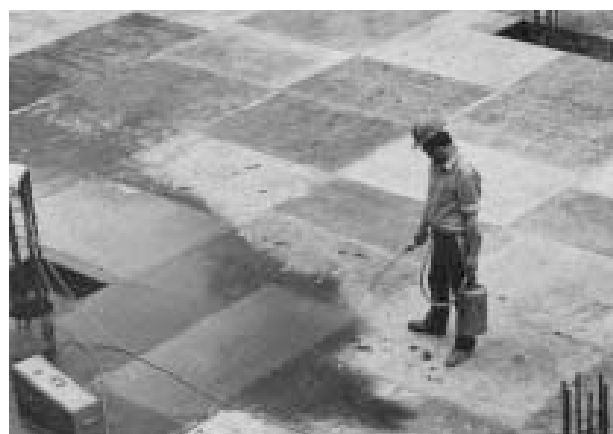
Figure 15.13 Release agent being applied to soffit form before reinforcement is placed
