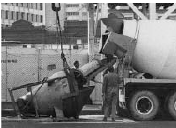
Figure 8.7 'Lay-down' crane buckets are easily filled from transit-mixers
