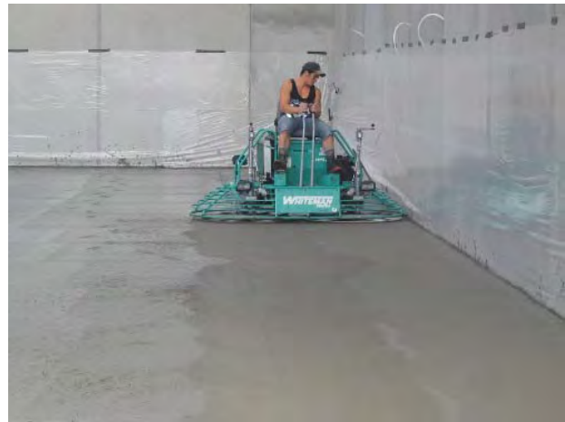
Figure 10.6 Ride on machine trowel
