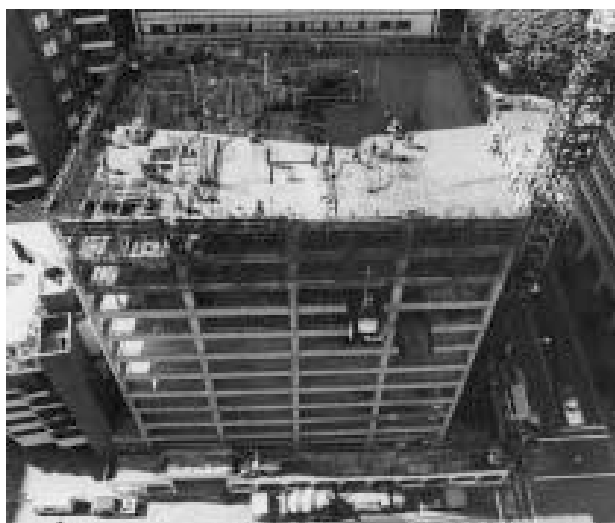
Figure 8.9 Concrete distribution by pump (from a discharge point in the street where permitted) is the most common method
