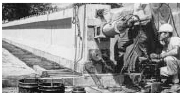
Figure 17.5 Post-tensioning jack operating on end of concrete girder
