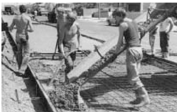
Figure 9.9 Use of an immersion vibrator at a slab edge
