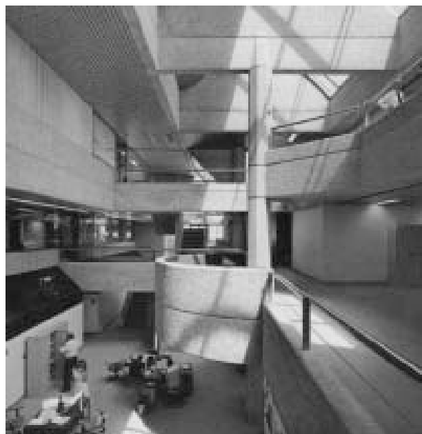
Figure 13.7 Example of bush-hammered finish which would require a test panel under NZS 3114 and AS 3610
