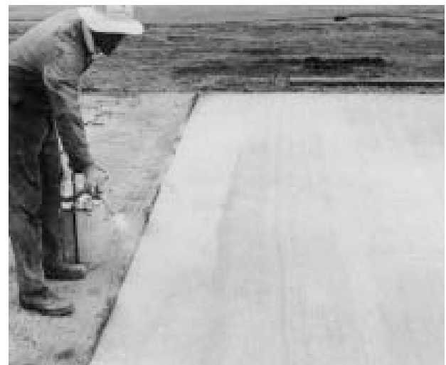
Figure 11.8 Spray application of curing compound
