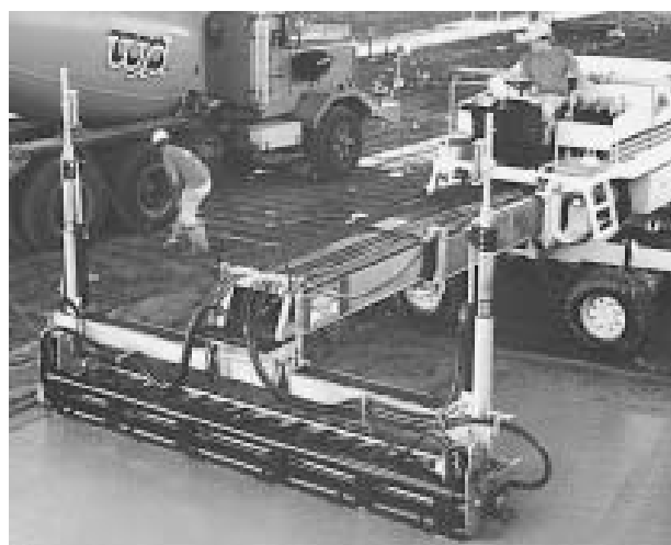
Figure 10.2 Typical machine-mounted beam screed
