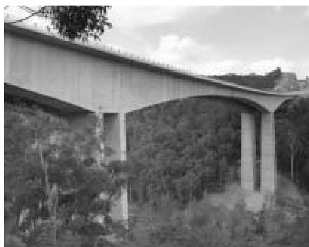
Figure 17.6 Multi-strand, post-tensioned bridge, Mooney Mooney, NSW
