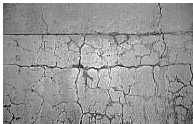
Figure 3.6 Typical map cracking caused by alkali-aggregate reactions
