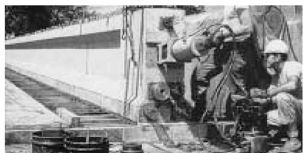
Figure 1.20 Post-tensioning jack operating at end of concrete girder
