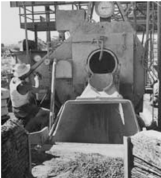
Figure 6.2 Typical small on-site plant with fan-shaped bins in front of a single hopper. (The large dial above the mixer indicates the weight of materials in the hopper, while the small dial near the operator is a flow meter indicating the amount of water.)
