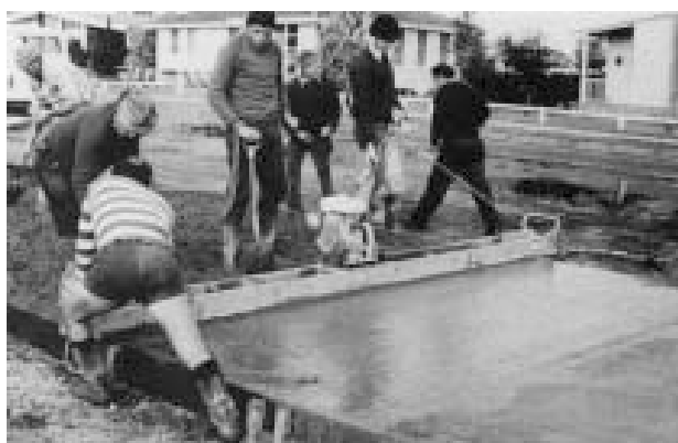
Figure 9.7 Typical screed vibrator
