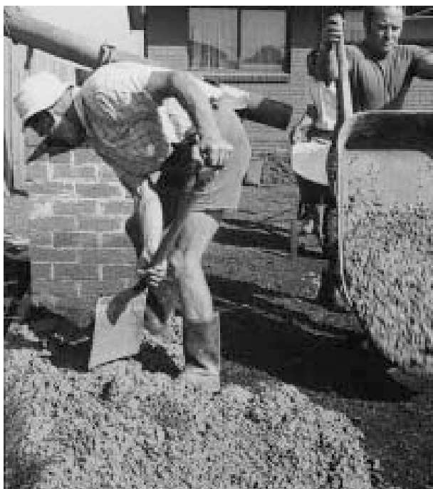
Figure 8.5 Barrows, despite their limitations, are the most suitable distribution means on small projects
