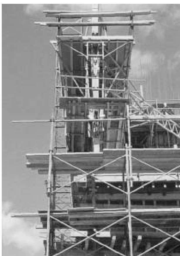
Figure 15.8 Slipforming a vertical element
